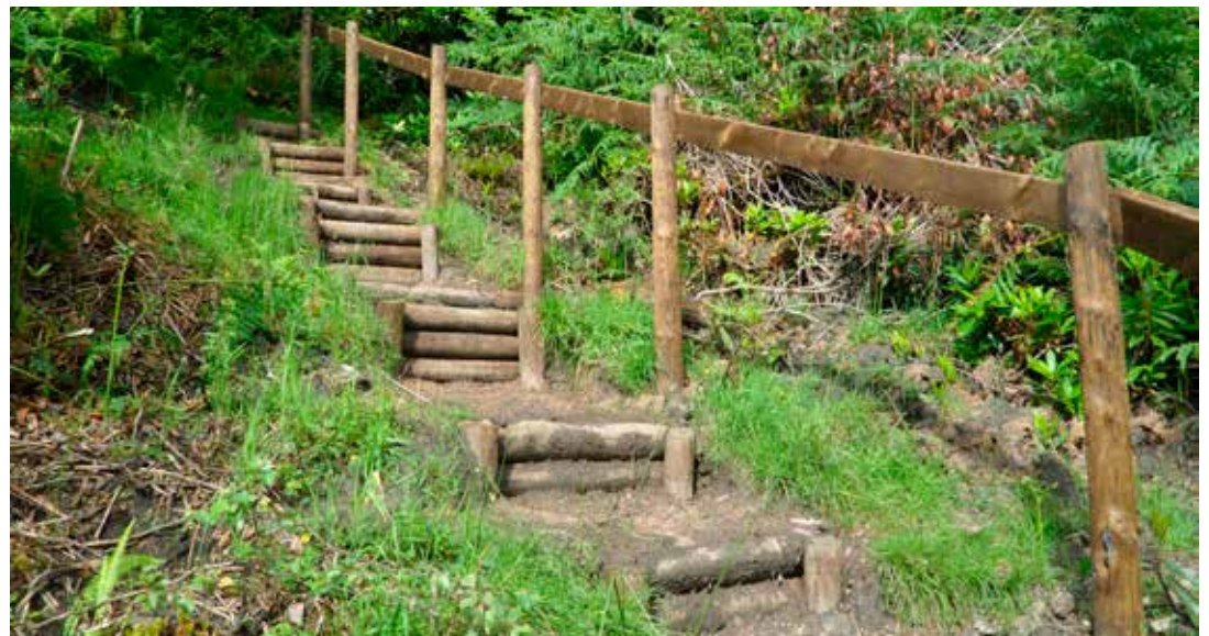
New wooden steps and railing at Ormidale Lodge
